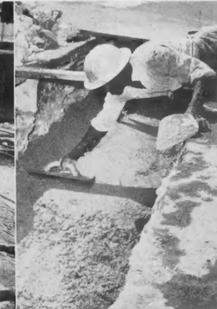
A GROUNDING system is installed by workers, above left. Others smooth poured cement before the ditch is filled, braze cables going through into the government substation grounding system, and build pull boxes through which Lago's power cables will be connected to government switching gear.
